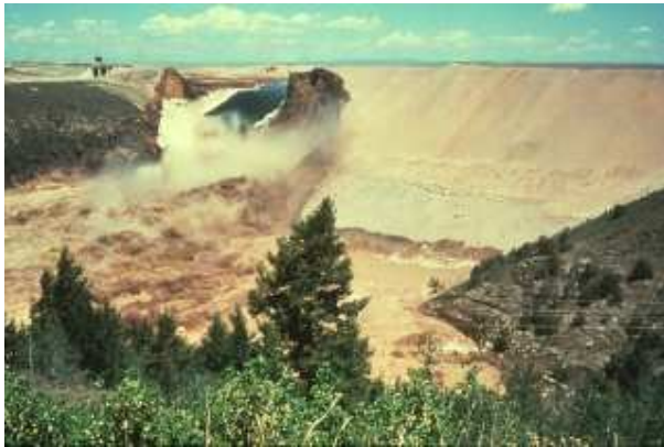
The Teton Dam failing, USA.
